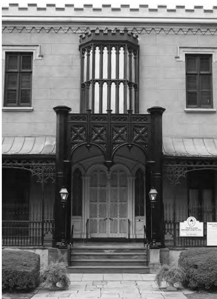
Doorway facing the garden of the Green-Meldrim Mansion
